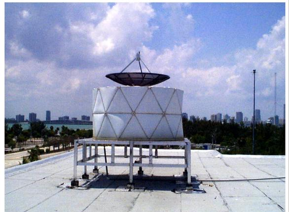
CoastWatch satellite antenna installed on the roof of the AOML facility (before addition of protective dome).
